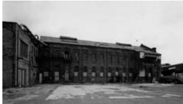
Fig 5. Original Ice Factory. Fox Street elevation of tank house with rear of 1950s compressor room on left. (NMR: AA006345)
