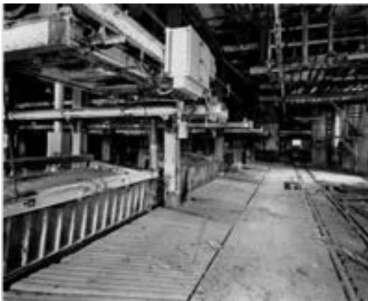
Fig 7. Original Ice Factory. Tipping cradles and distribution area on ground floor of tank room. (NMR: AA006374)
