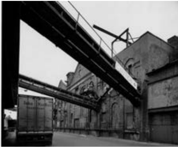
Fig 4. Original Ice Factory. Gorton Street elevation of tank house and ice store. (NMR: AA006353)
