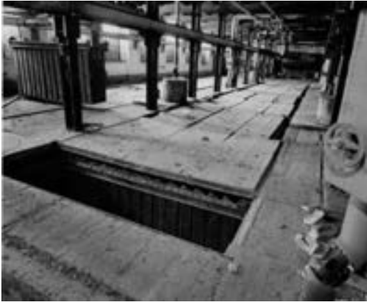
Fig 6. Original Ice Factory. Ground floor of tank room, from NE. (NMR: AA006371)
