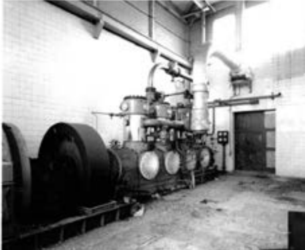
Fig 15. Interior of 1950s compressor room from SW. (NMR: AA006394)
