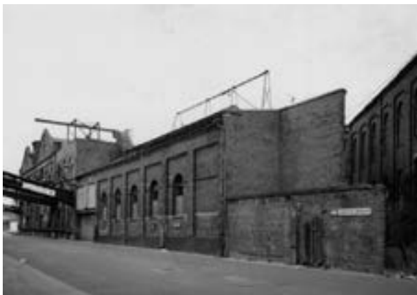
Fig 10. Original Ice Factory. Boiler house and site of chimney from NE with tank house and ice store beyond. (NMR: AA006354)
