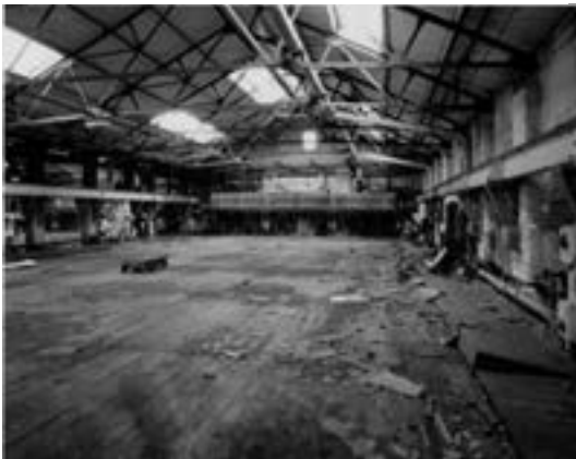
Fig 8. Original Ice Factory. First floor of tank house from NE. (NMR: AA006384)
