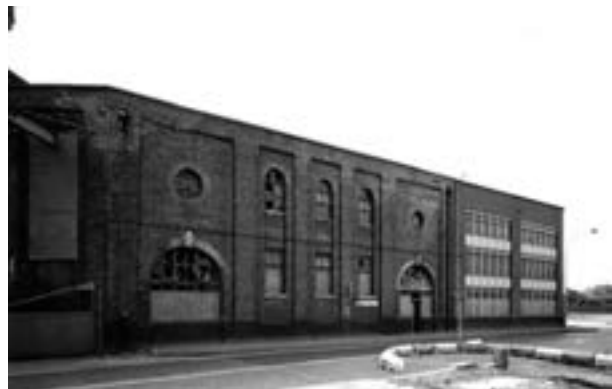
Fig 11. Original Ice Factory. Exterior of compressor house from NW. (NMR: AA006358)
